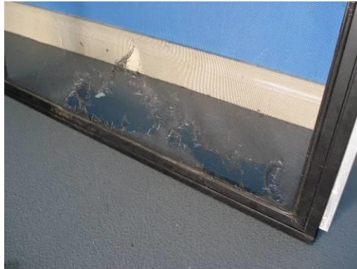
Doorway and flyscreen damage caused by a pet
